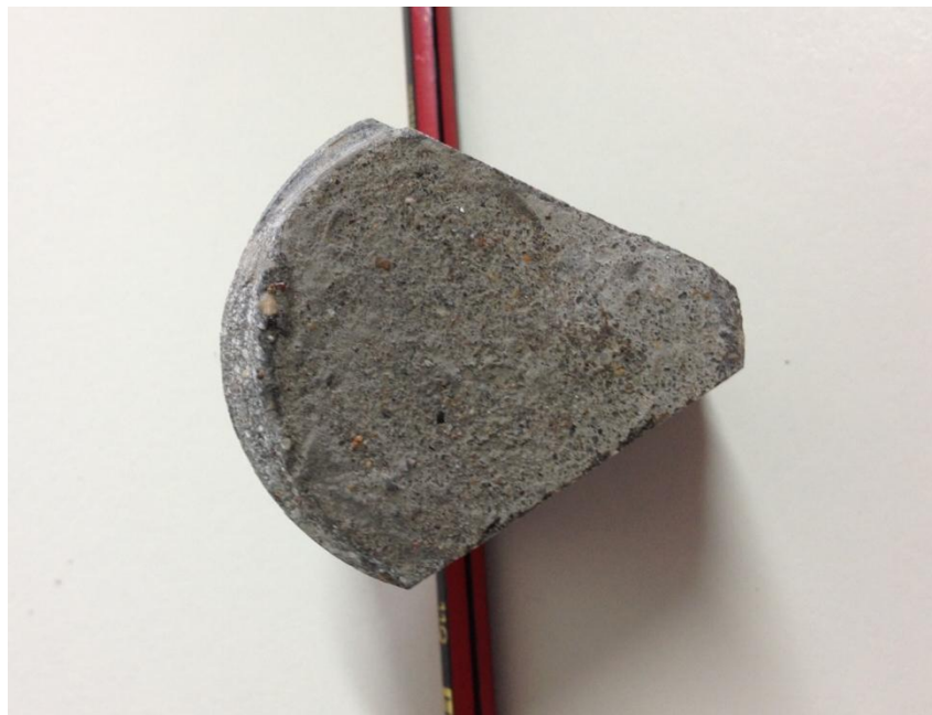
Photo 5: Core top surface after removing Faux Brick on two edges
