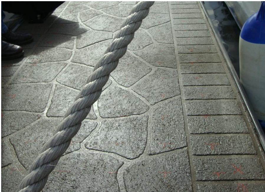
Photo 3: A closer view of the jetty slab top surface condition
